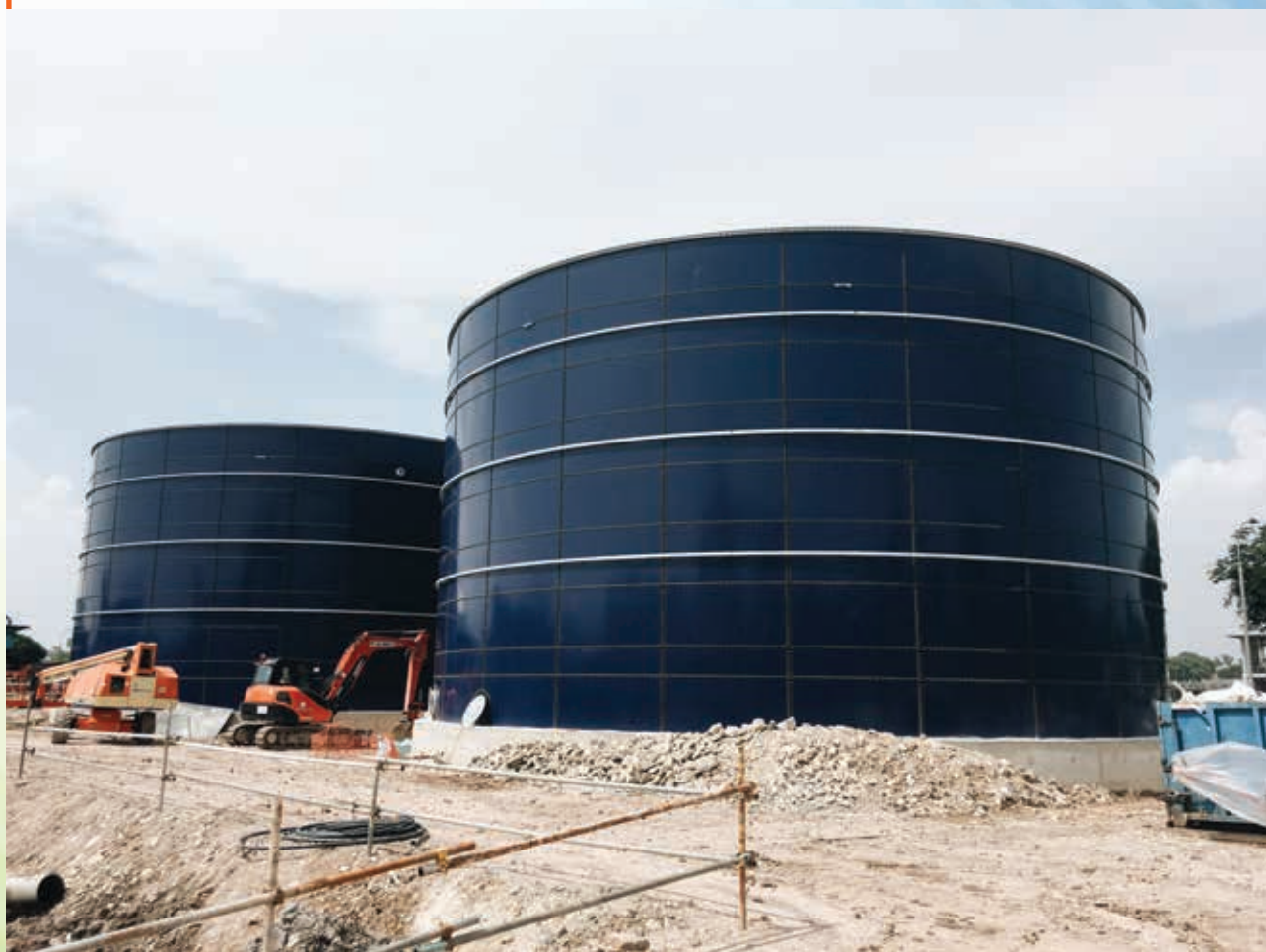
JURONG WATER RECLAMATION PLANT – bolted steel tank
